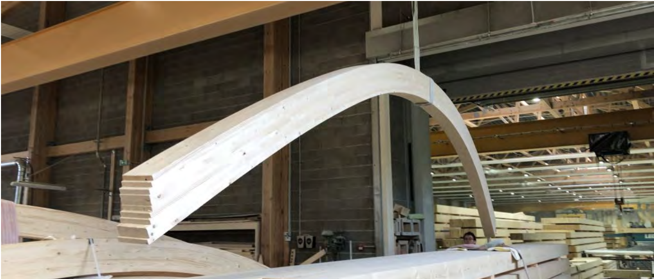
Fabrication of a curved glulam member.
