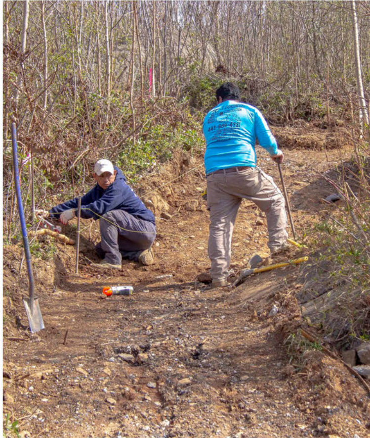
Construction lines being established for a raised path built with on-site construction
