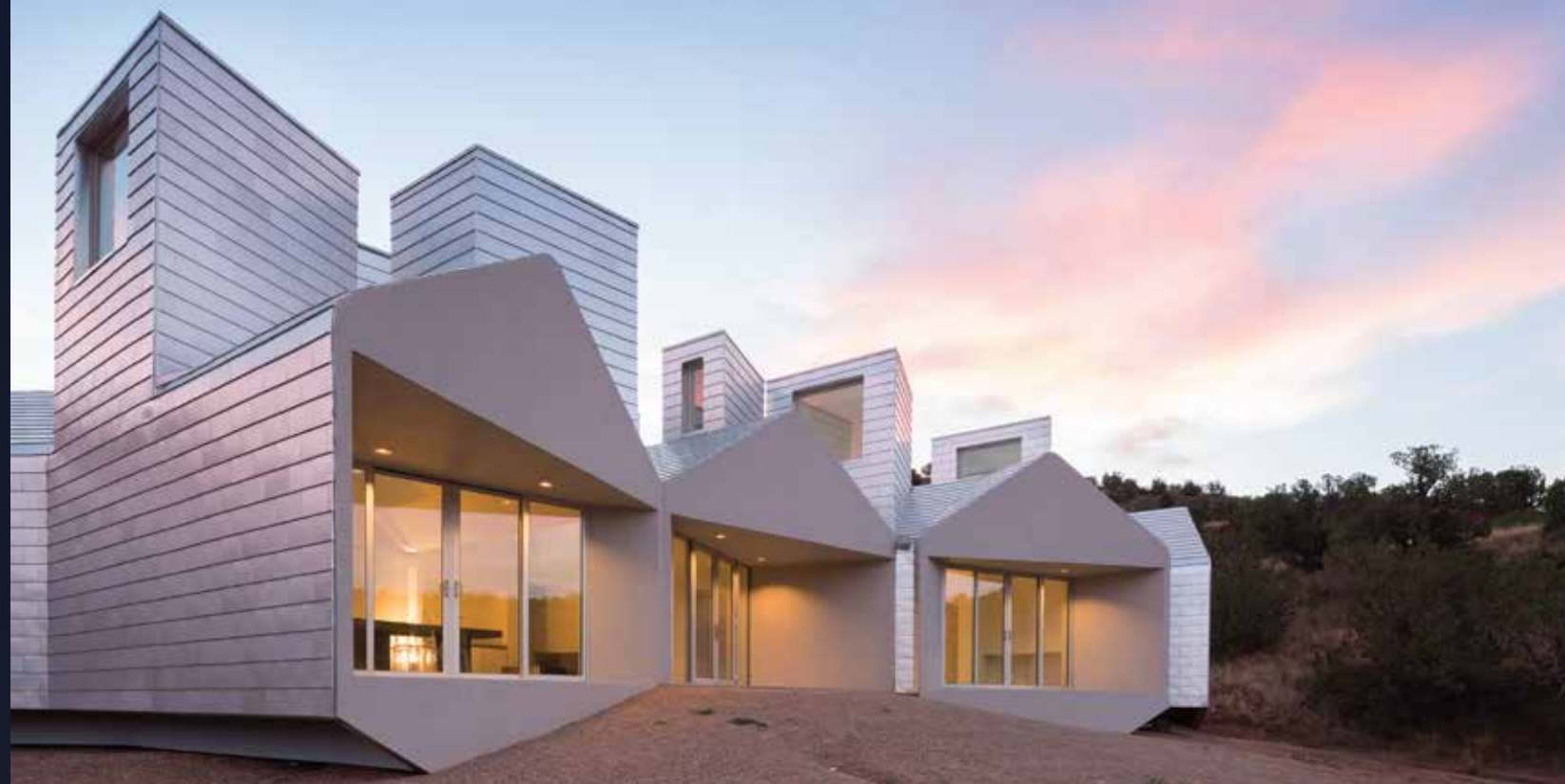
Element House was commissioned by the Museum of Outdoor Arts and designed by MOS Architects. This prototype was constructed to serve as the guest house to visitors of the earthwork, Star Axis , by Charles Ross in New Mexico. Photo by Florian Holzherr.
